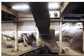
BLUES Anlage in Schorn
